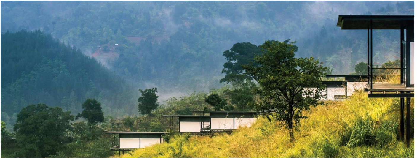
Villas built on undulating terrains overlooking the environment.
