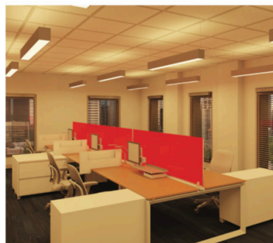
Example of tuned luminaires in a work space that deliver extra CS to a space's occupants (LRC, 2016)
